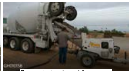
Concrete truck and line pump
