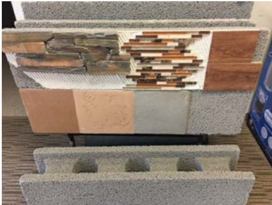
(Figure 9.5) Photo of a display, illustrating faux stone and tile applied directly to the block with Thinset mortar. The block just below, shows the bare block (illustrating the texture of the face of the block), a stucco "brown" coat (actually gray in color) applied (keyed) directly into the block texture, and two different examples of finish coats (Monterey and Sand finishes). These applications on bare ICCF block require no additional layers of foam or chicken wire (lath) and tar paper, saving material and installation costs.
