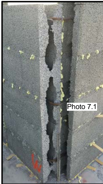
Photo 7.6a Tack gluing (every 12") of the first course.
