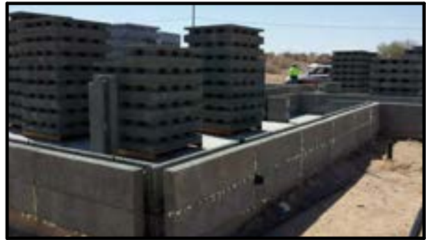
Photo 7.8 The second course placed, plumbed, leveled, and glued. (10" Asymmetric Block pictured)
